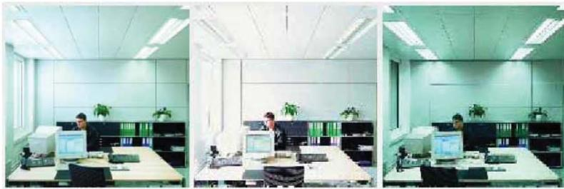
Fig. 52: In the morning, no light is needed from the row of luminaires near the window.
